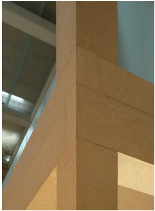
Corner intersection of the precast construction in the Egyptian Courtyard
