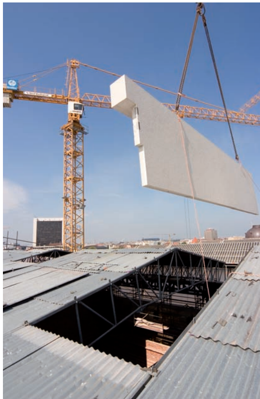
Lifting a precast element through the open temporary protective roof
