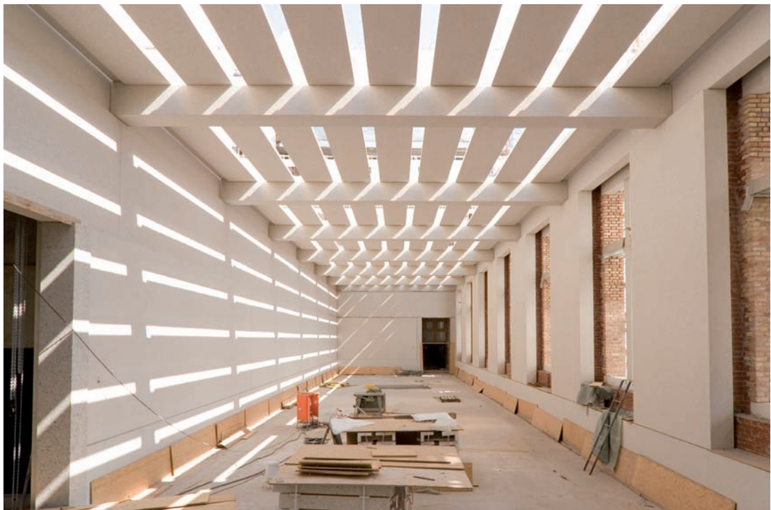
Rolling ceiling in the assembled condition without upper ceiling and with still open intermediate spaces
