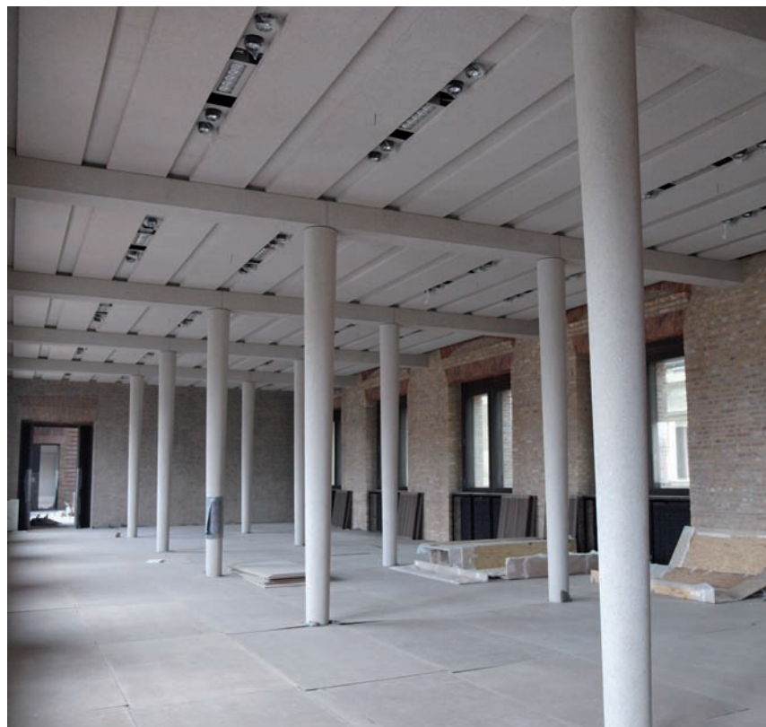
Finished rolling ceiling with built-in lighting units and 'carrot columns'
