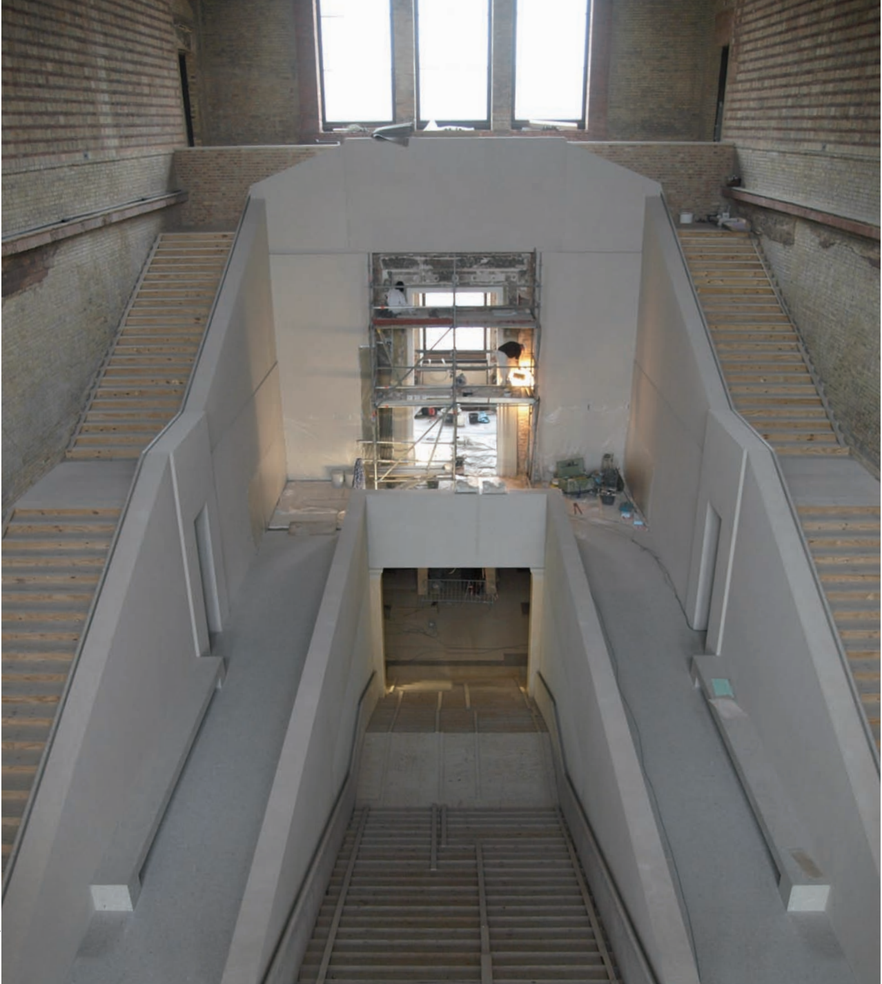
Main staircase with new stairs made of high quality architectural concrete
