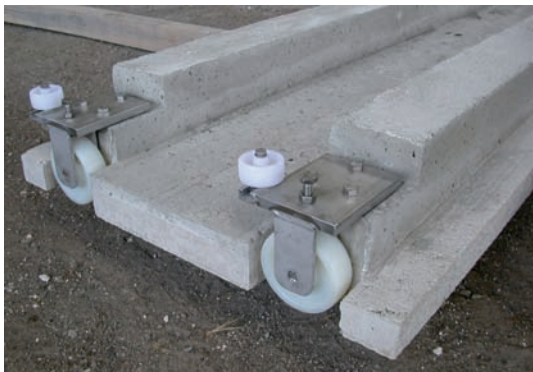
Rolling mechanism for the suspended ceiling
