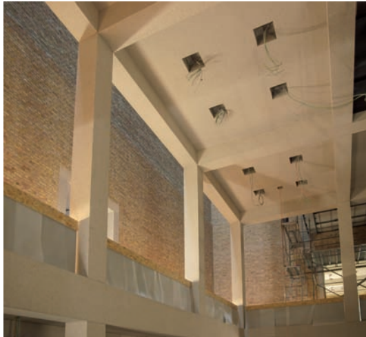
View of the precast platform in the Egyptian Courtyard from below
