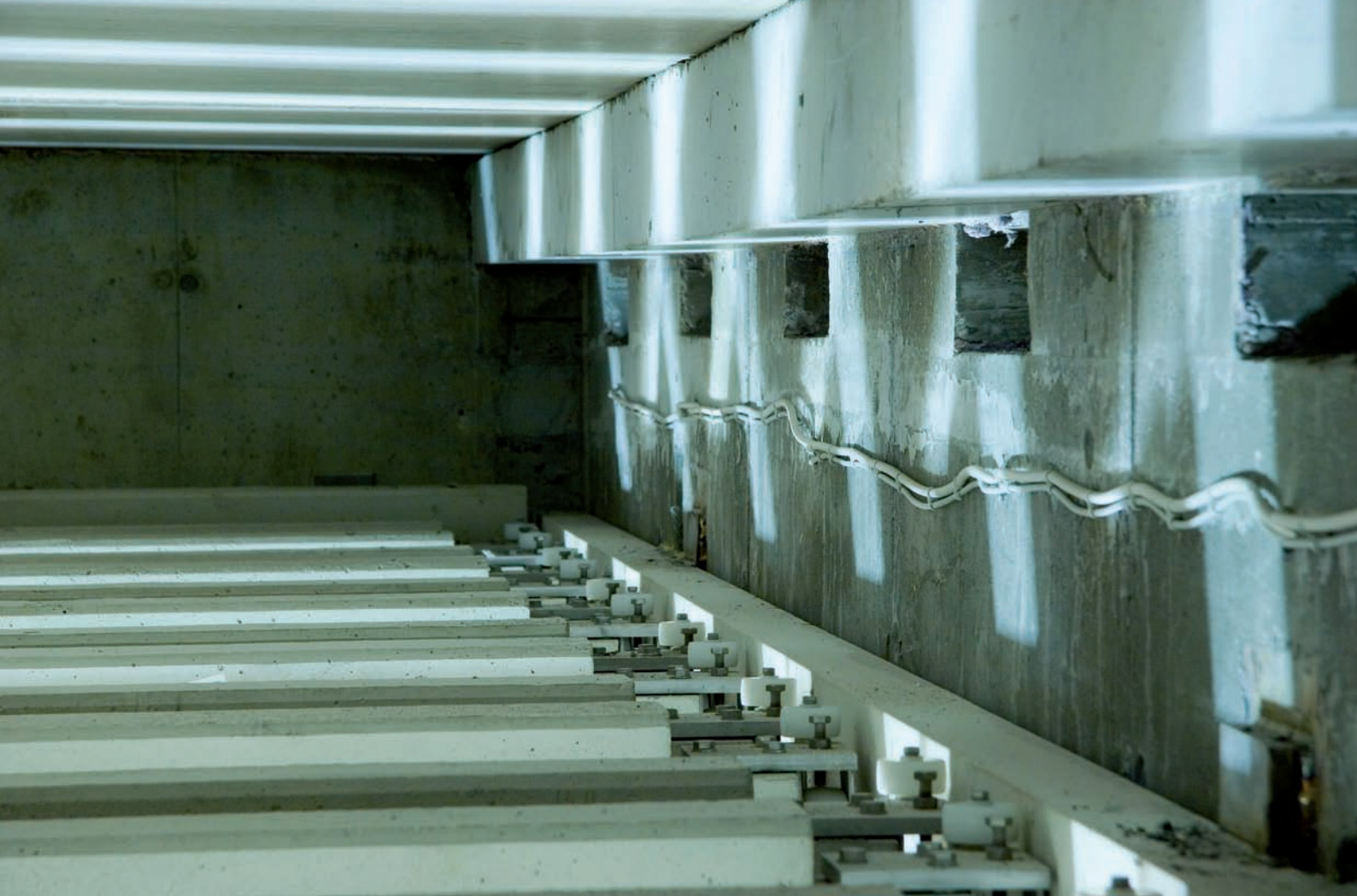
Intermediate space between the suspended ceiling and the supporting storey ceiling
